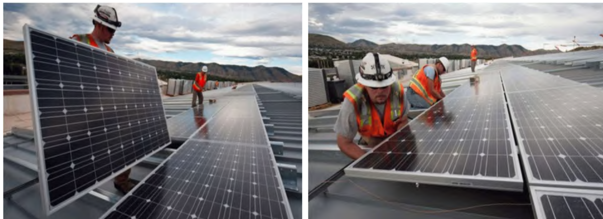
Figure I-11 Installation of a nonresidential CSPV system
